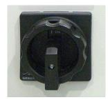
The main switch is on the control cabinet of the system.
