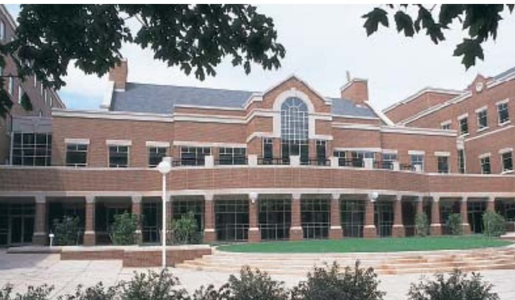
Common spaces in the new Advanced Technology Research Center, dedicated Oct. 11, will facilitate interaction between students, faculty and engineers from industry, cutting across the lines of traditional academic disciplines.
