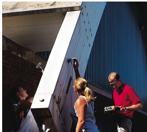
The Colvin Center Annex is the site for graduate student Sarah Markes' thesis project. Under the tutelage of Robert Emerson, an assistant professor who joined the School of Civil and Environmental Engineering this past year and specializes in timber structures, Markes is evaluating decay in the beams that support the facility's roof. The study involves using non-destructive means - ultrasonic wave inspection in this instance - to predict the internal condition of timber. Undergraduate Jennifer Prichard (left) sends a wave through the beam that Markes captures with a transducer while Emerson records the time duration.
